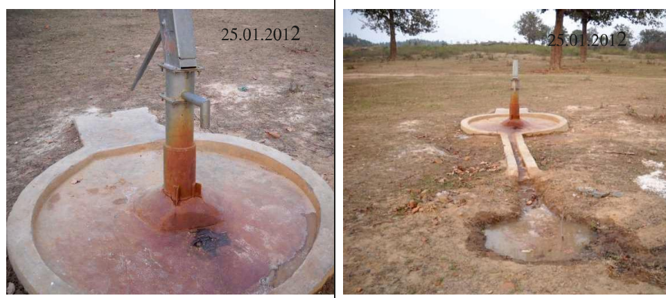
Photographs showing reddish platform of hand pumps due to high content of Iron in water at a village in Block Sitapur, District Korea
