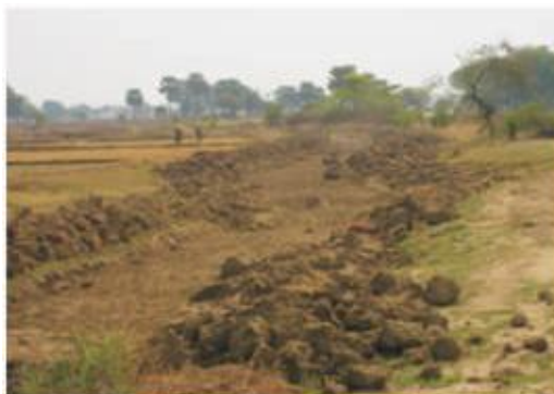
Scheme No. 17/11-12 Chahaka (Karha) was digging only in 11000 cft(1100'x10x1'), whereas 40955.79 cft work was shown in the MB.(GP-Baligaon, Rafiganj)
