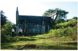
Incomplete earth work for bridge approach without any retaining wall and protection work on Simaluguri side.
