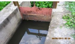
Fully closed Cross Regulator of the Headwork Head Regulator at the Headwork (6 May 2013)
