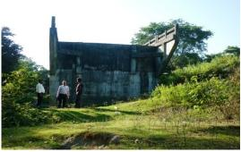
Incomplete earth work for bridge approach without any retaining wall and protection work on Simaluguri side.
