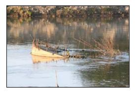
SHIFT AND TILT OF SUBMERGED PIER NO.1 (26/12/2011)
