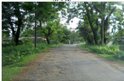
ROAD FROM MISAMARI CENTRE TO MAILBAGZAR VIA GOMIRI CENTRE (CH 430 M) (29-5-12)
