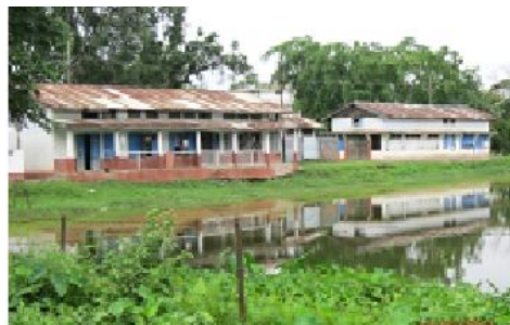
Two buildings training centre, Joysagar occupied by Army (June 2012)
