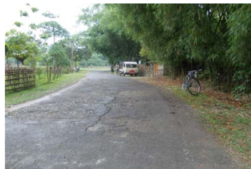
IMPROVEMENT OF KAMARGAON ALI ROAD (CH 1,230 M TO 1,290 M) (2-6-12)
