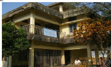
Idle building at RFTI, Amranga occupied by army (February 2011)
