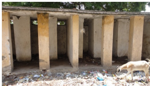
Toilets at Konapapet shelter in East Godavari District
