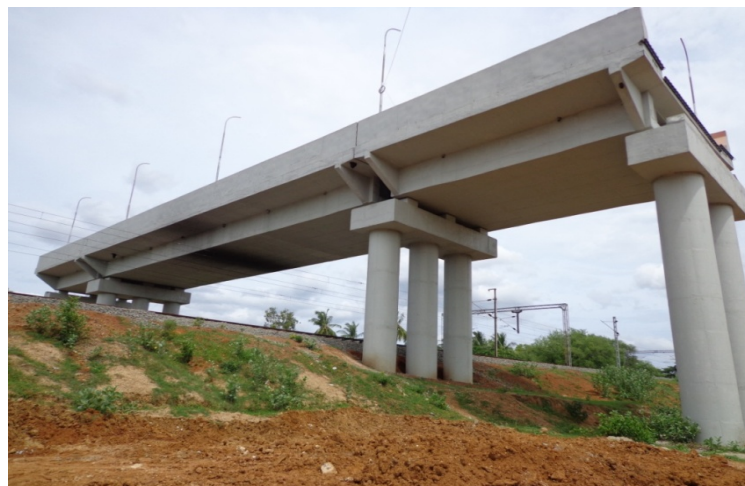
Bridge proper at Tummikapalli completed, but approaches incomplete
