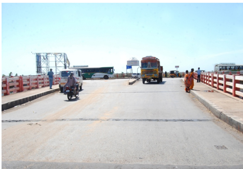
Direct traffic (bus) forced to take elevated T-junction at ROB at Kovur Gate
