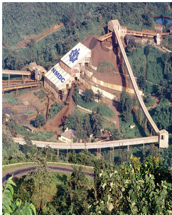
Fig 2: Aerial view of downhill conveyor at Bacheli
