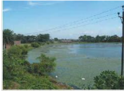
BSUP Phase-IV project ,Patna, Bihar – Abdul Rahmanpur site low lying area litigated & submerged under water (BSUP Project, Bihar)
