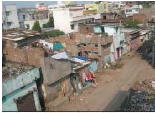
BSUP Phase-IV project ,Patna, Bihar – Salempur Dumra Site occupied by Private Building
