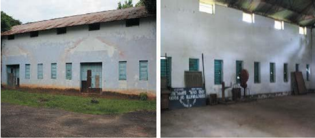
Departmental State godown (500MT) at Dimapur Photograph dated 25.7.2011
