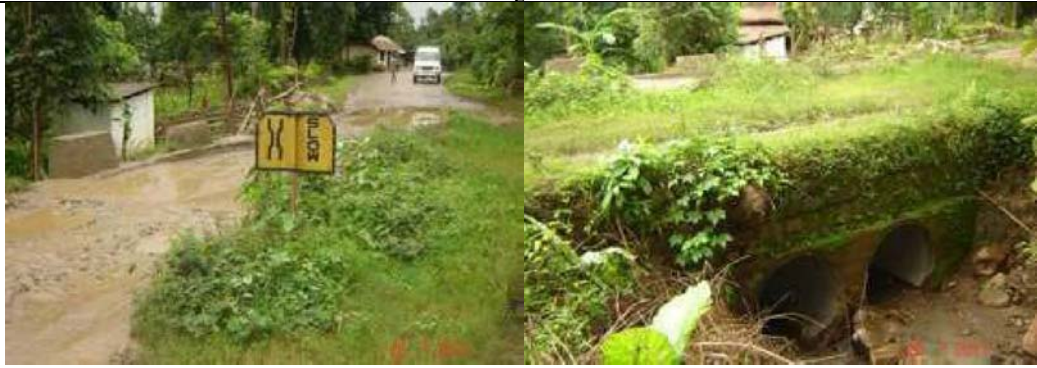
Incomplete RCC slab culvert at Socunoma village on Medziphema-Jalukie-Athibung road
