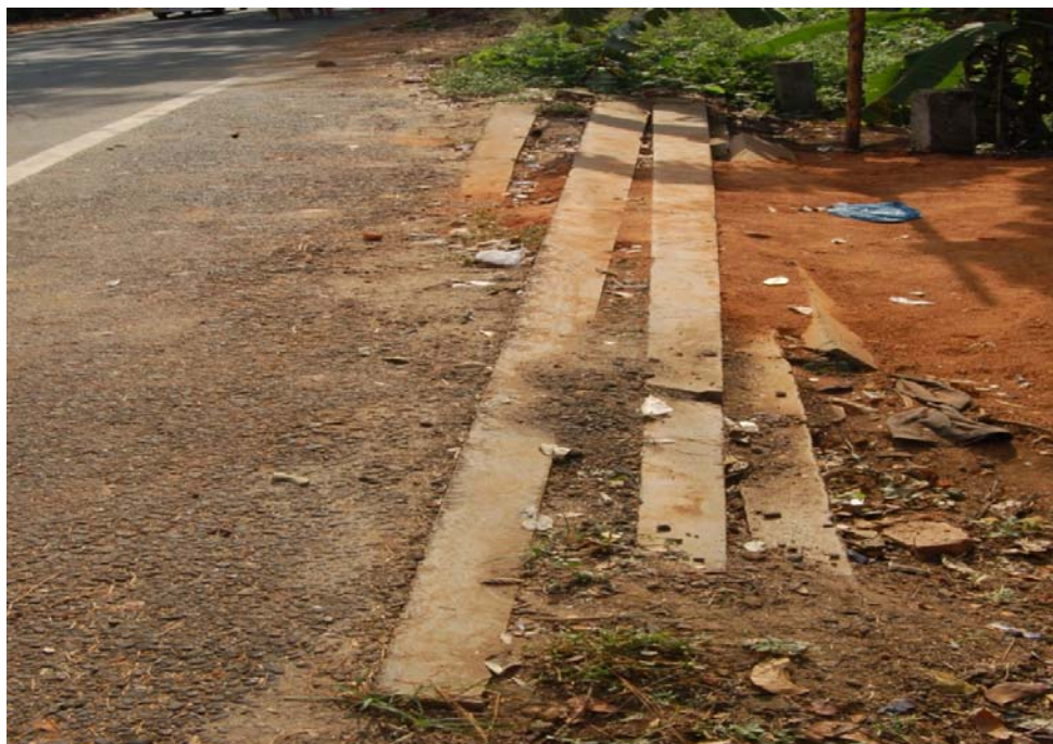
Poles stacked on way side and buried under soil and bitumen at Thodupuzha EC.
