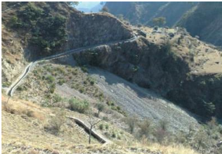
Uncovered hydel channel: Hydro Power Project Manjhal, Chamba District (Photograph dated 10 April 2012)
