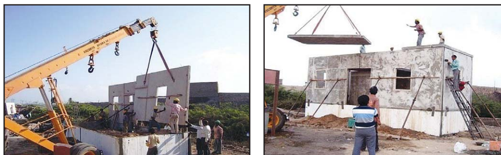
(Picture showing erection of precast panels for CCP/COP)
