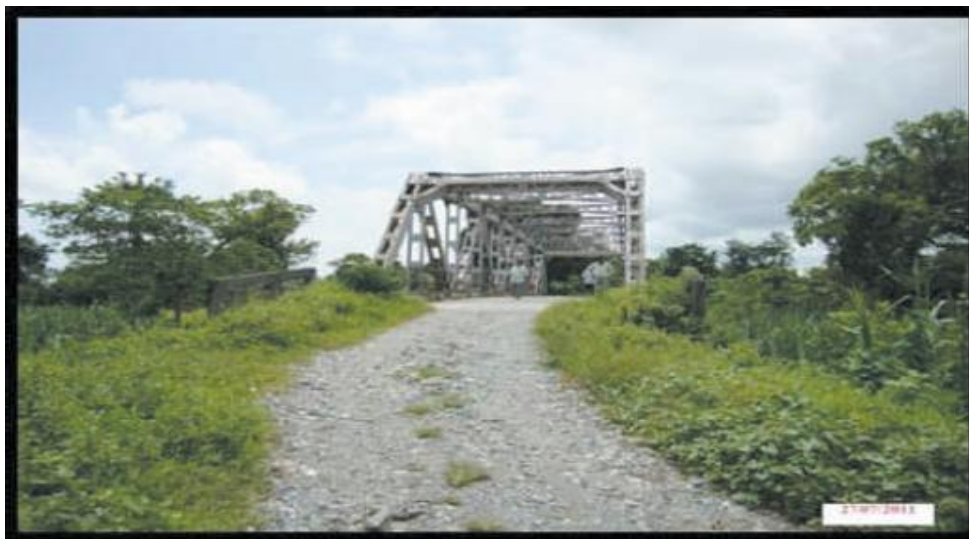
Steel Bridge over Kundil River between Iduli and Kabang Village
