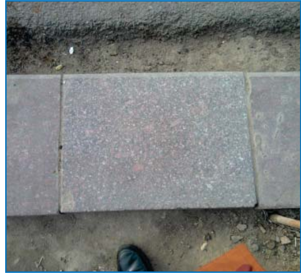
Granite kerb fixed at work site
