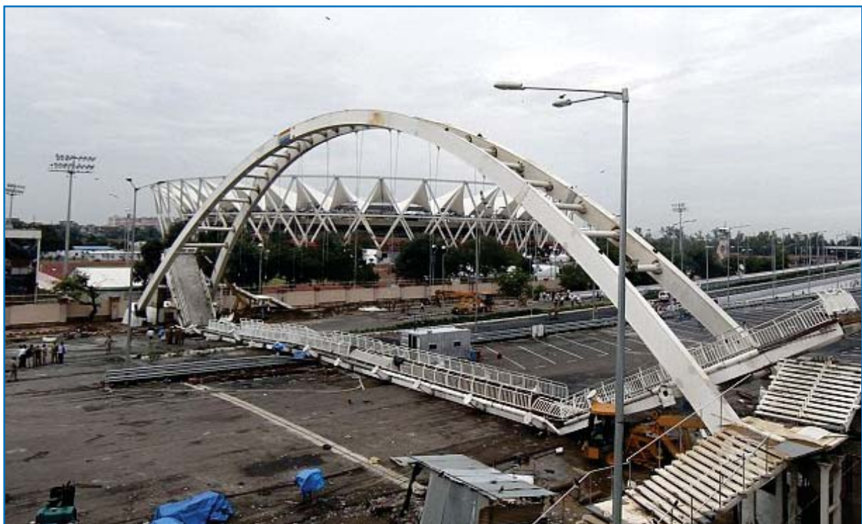
Collapsed FOB near JLN Stadium
