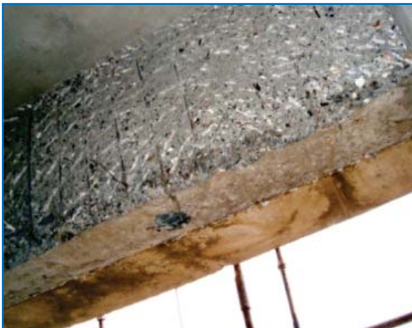
Chipping of beam (Report No. 9-Tower 1)
