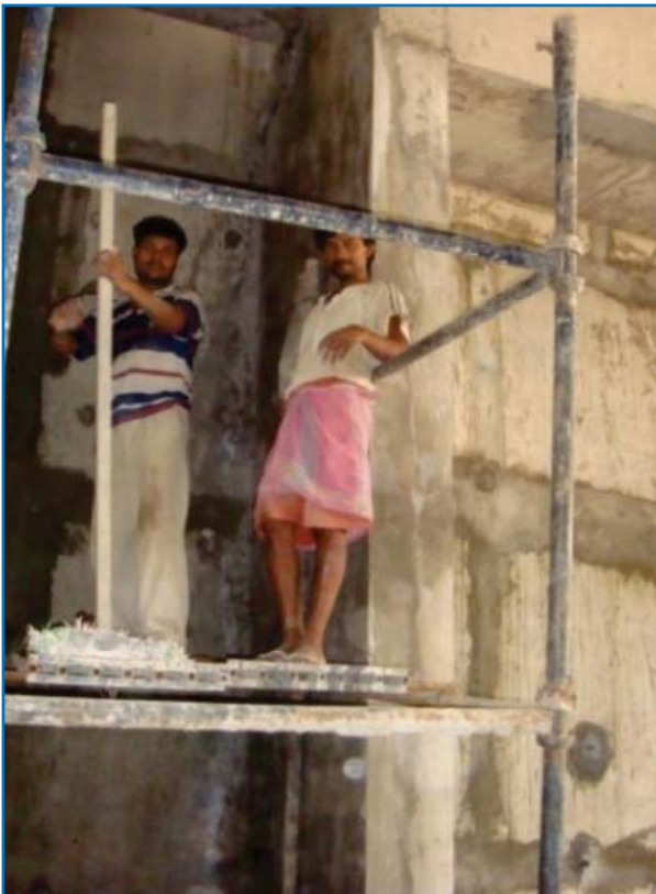
Plastering of defective column in Tower-5 (Report No. 3)
