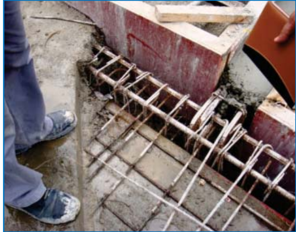
Concreting was in progress without bending reported in CBRI Report No. 4
