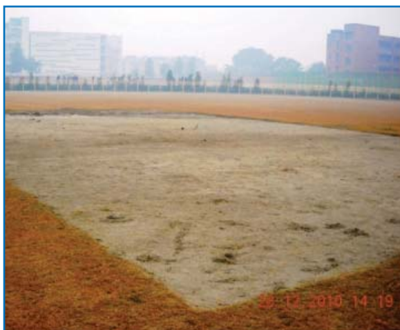
Restoration work of cricket field in Rugby 7s training venue
