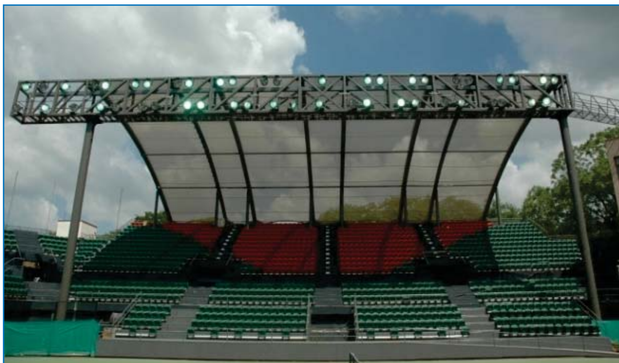
Centre court after renovation
