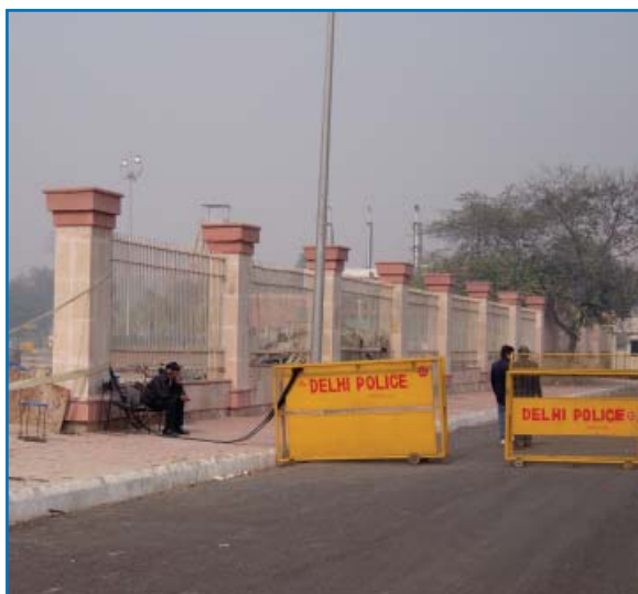
Boundary wall between Gate No. 9 and Gate no. 10
