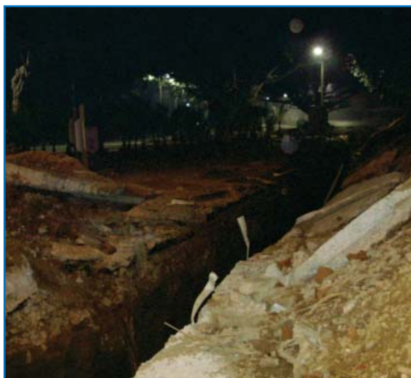
Digging work still in progress (Dec. 2010)
