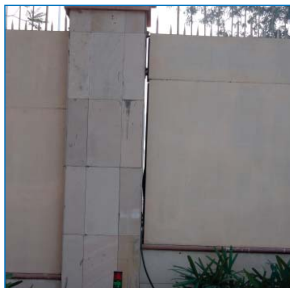
Gap in MS Plate security cover
