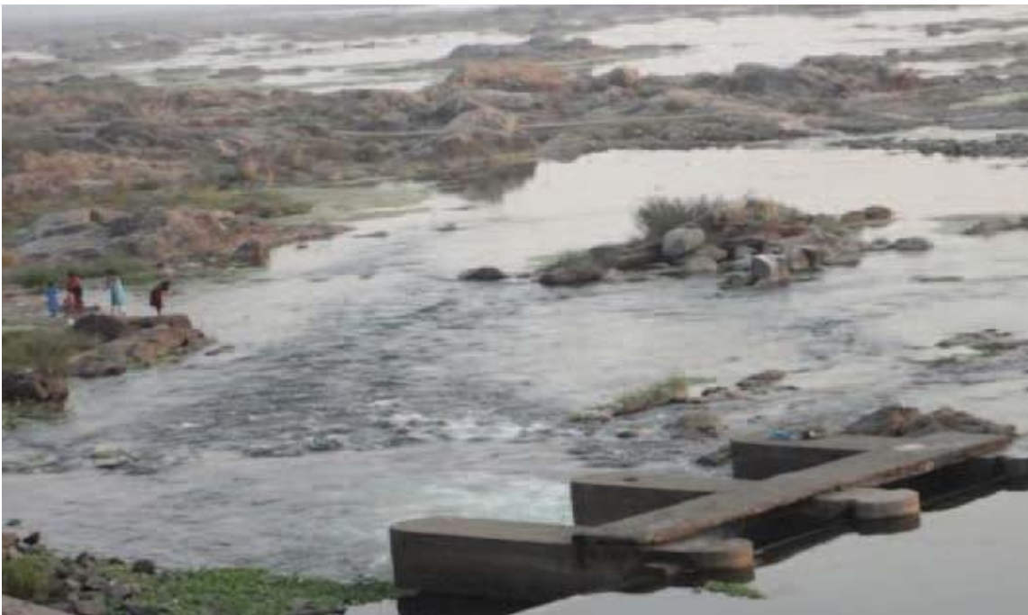
Untreated sewage flowing directly from STP into Bay of Bengal in Puri
