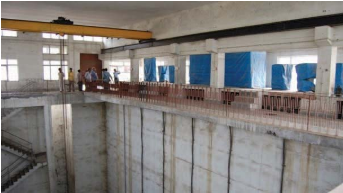
Incomplete Intermediate Pumping Station at Munsipurwa, Kanpur
