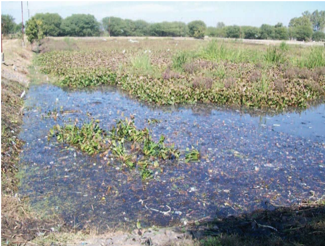
Sewage accumulation due to waste stablisation pond not being cleaned in for STP, Kshipra River, Ujjain
