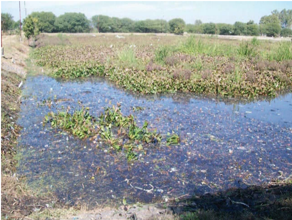
Sewage accumulation due to waste stablisation pond not being cleaned in for STP, Kshipra River, Ujjain
