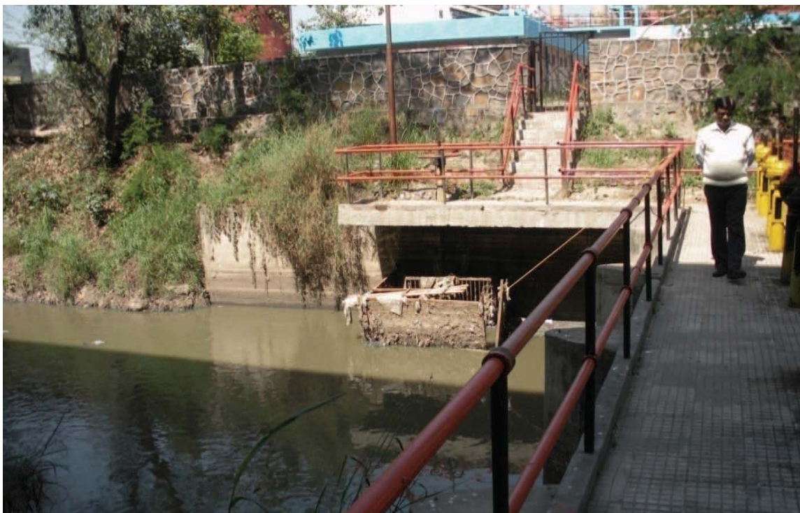
10 mld STP at sen Nursing Home (untreated sewage flowing to yamuna)
