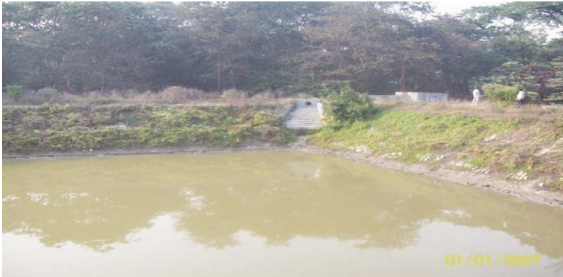
Non functional STP at Halilshar
