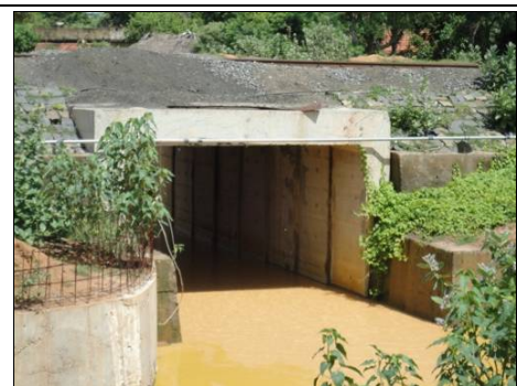
Water stagnation at an incomplete LUS site near LC No.189 in VM-TPJ Sn.(SR)
