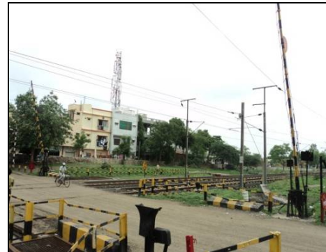
LC No.1B at Nagda (WR) not closed even after commissioning of ROB
