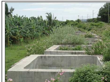
Cast RCC boxes for LUS lying idle at unmanned LC No.4 in CGL-AJJ Sn.(SR)
