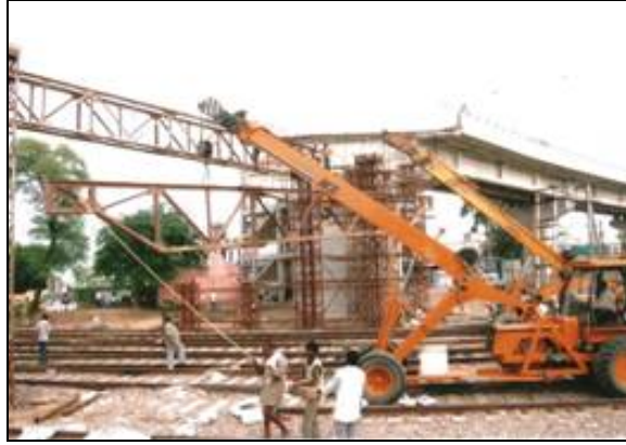
ROB work at LC.No.57-B (Rewari) sanctioned in 2003-04, still in progress (NWR)
