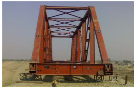
Open web girder
