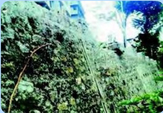
Protection for houses above the road
