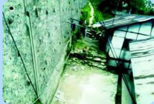
Protection for houses below the road
