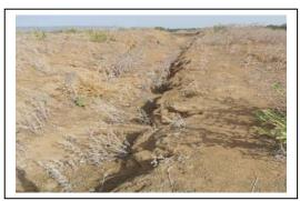
Water course filled with silt and sand in Chak  $M_2S_2L_5$
