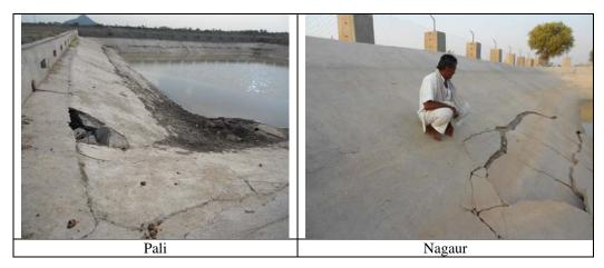
Photographs showing defective water sources with leakage/cracks (Pali and Nagaur)
