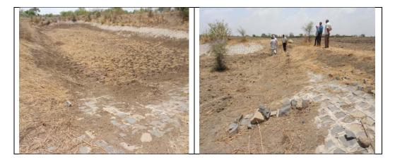
Photographs showing defective and mud filled water sources with broken sides - Jhalawar
