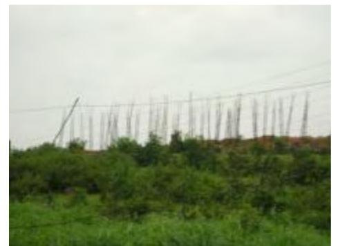
Abandoned administrative building at IRBN, Koraput
