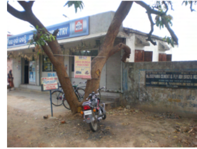
Use of land for partly commercial purpose though leased for industrial purpose (Seepona Cement and solid Brick), Paramanandapur, Kalahandi District
