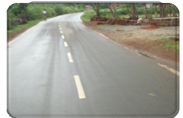
Portion of New Jagannath Sadak in Trafficable condition - 67.60 km Picture No.2.4.3
