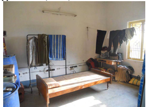
CIPA II infrastructure used as a rest room at Chandili PS of Rayagada district
