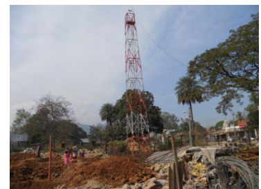
Abandoned MART Towers at Muniguda PS of Rayagada district
