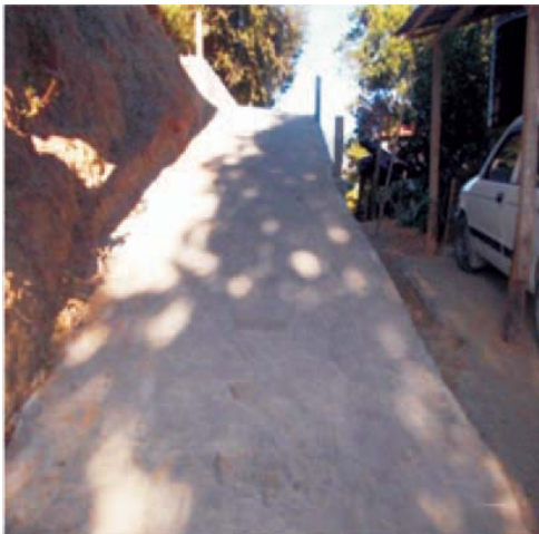
A photograph showing Construction of Stone Masonry steps with masonry pavement alongwith hand railing near Chawngkunga garage to Nunzami house, Luangmual (no hand railing provided)
