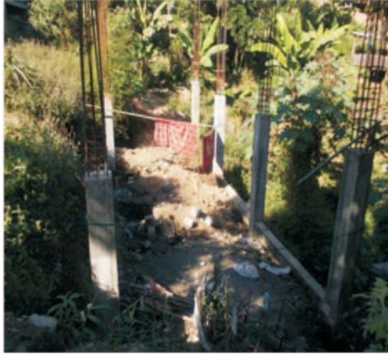
A photograph showing incompleted status of Construction of Community Hall, Phungchawng.
