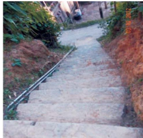
A photograph showing Construction of Stone Masonry steps with chequered tiles from Mawitea's house to K. Lalrinzuali's house, Luangmual (no chequered tiles provided)
