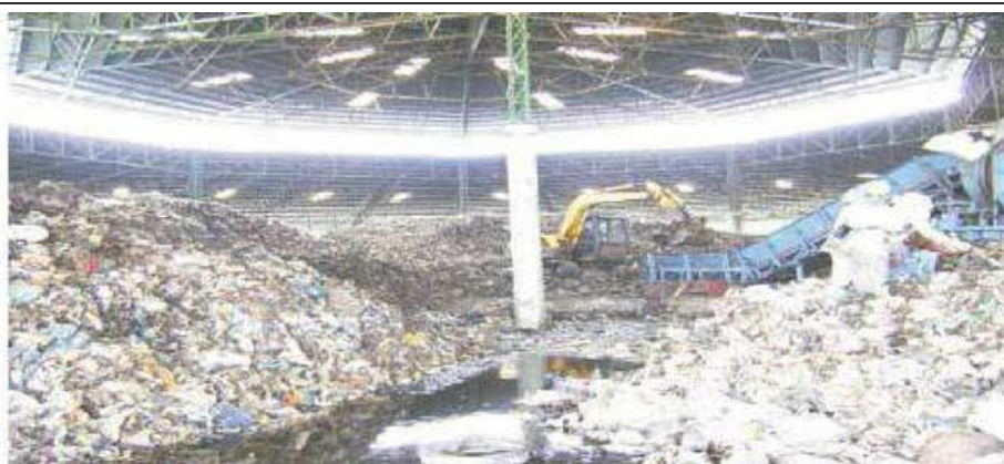
Un-segregated solid waste at Mawiong Compost Plant
