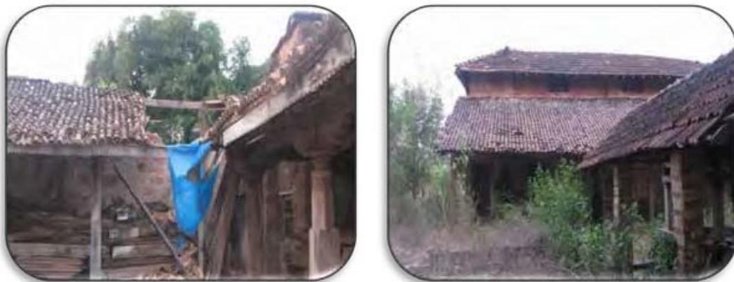
Portions of roof and a wall inside the palace had collapsed and some of the wooden planks had bent on account of usage of heavy weight bricks during conservation. Government stated (December 2011) that further conservation
