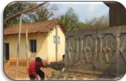
Rameshwara Temple Chittur, Soraba taluk, Shimoga district with an Anganawadi Centre in front of the monument
