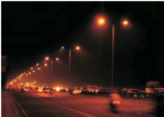
Modernised Street Lighting in Delhi
