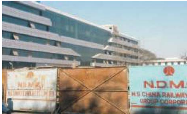
Barricading in the names of main/sub-contractor at worksite
