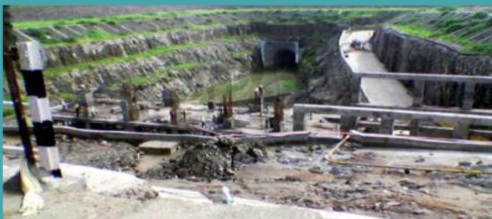
Indira Sagar Project (Canal) – Madhya Pradesh : Punasa Exit Channel – Work in Progress
