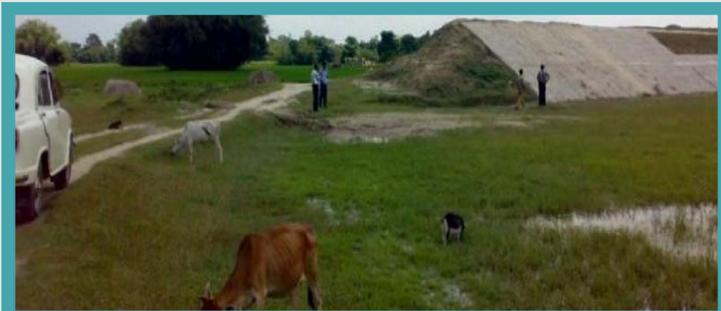
Teesta Barrage Project - West Bengal : DNMC of TBP at Ch. 63.585 where no trace of canal water was observed due to land dispute in Uttar Dinajpur District
