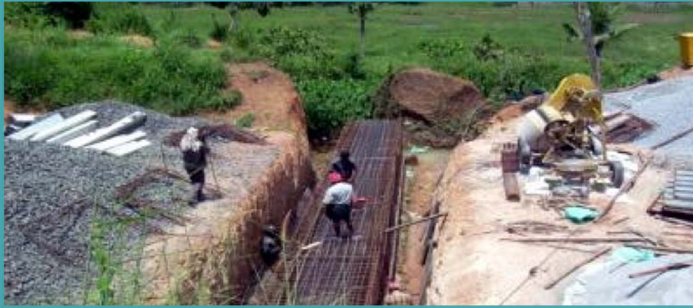
Kallada Irrigation Project - Kerala : Poovattoor Distributary-Bottleneck work in the Railway portion – Work just started
