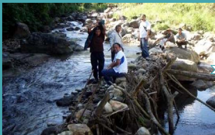
Damaged headwork at "Improvement and Renovation of Sipir MI Project" at Ayang Village, Pasighat Division
