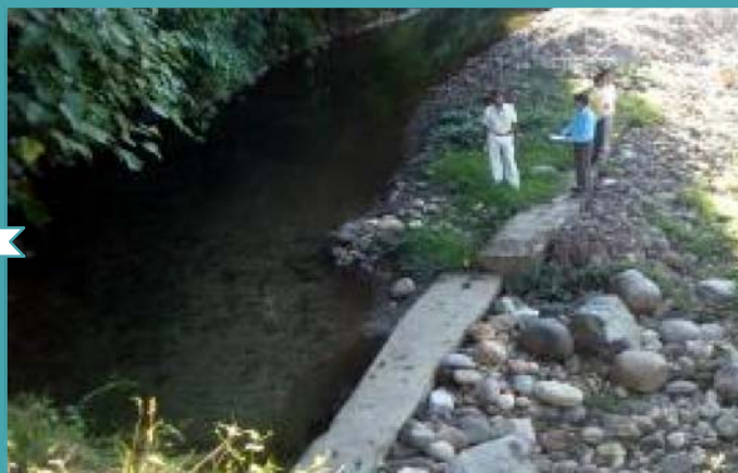
Completely damaged headwork at "Renovation of Headwork of Gagur MI Project" at Niglok, Pasighat Division
