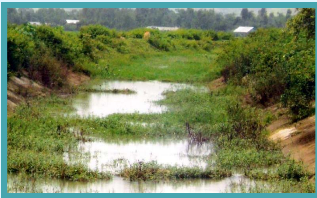
Thoubal Multipurpose Project - Siltation & shrubs/ weeds in canal
