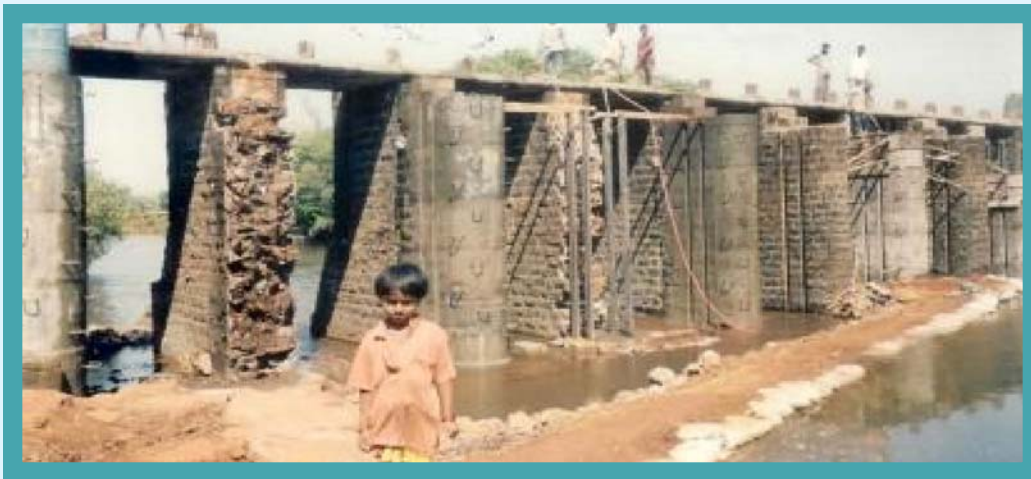
Repairs to the existing KT weirs in Patgaon Medium Project yet to be carried out
