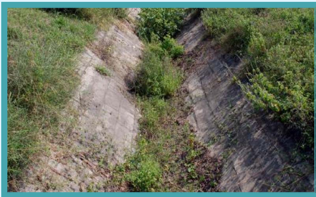
Mukteshwar Project-Dry canal with Weeds and Siltation
