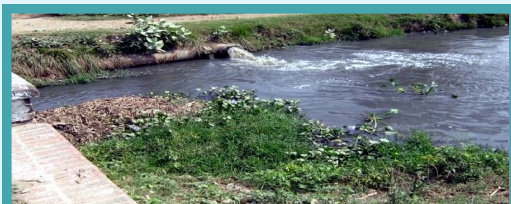
Discharge of Sullage/Polluted water at RD 58500 metre of Chheharata Distributary of Upper Bari Doab Canal (UBDC)
