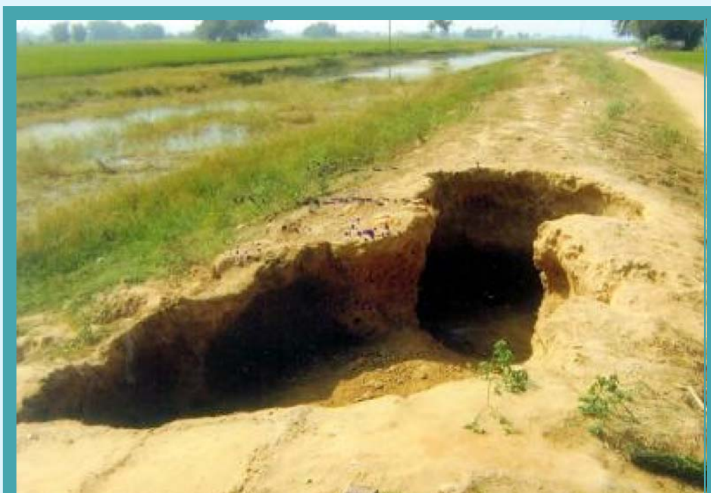
Damaged embankment of Gerua Reservoir Scheme
