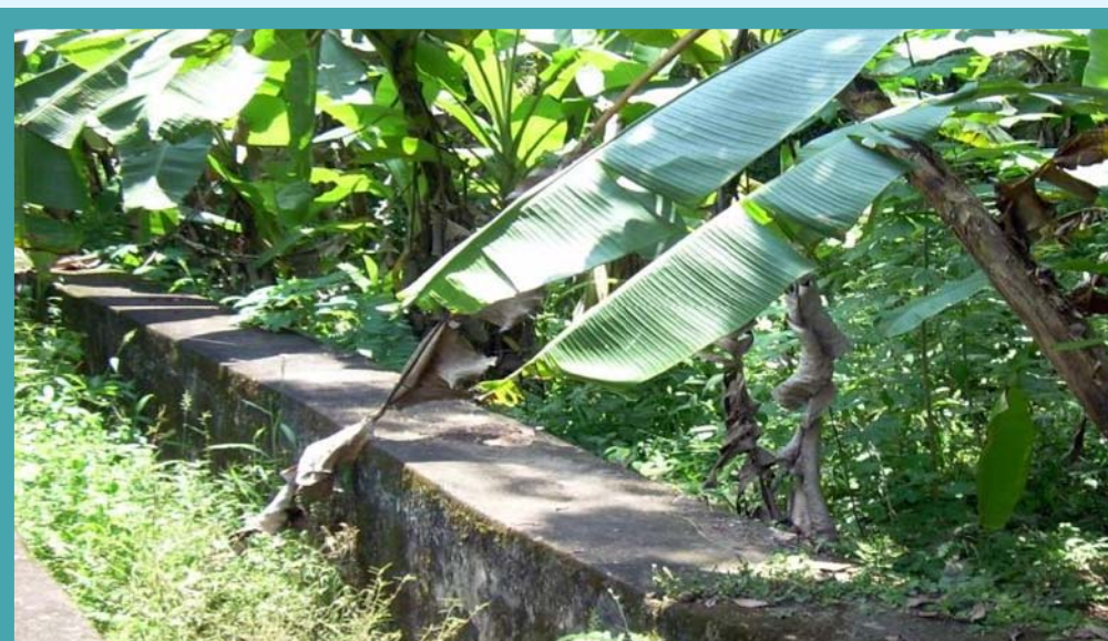
Pulamon Distributary of Kallada Irrigation Project – Canal filled with grass and plantations on the banks
