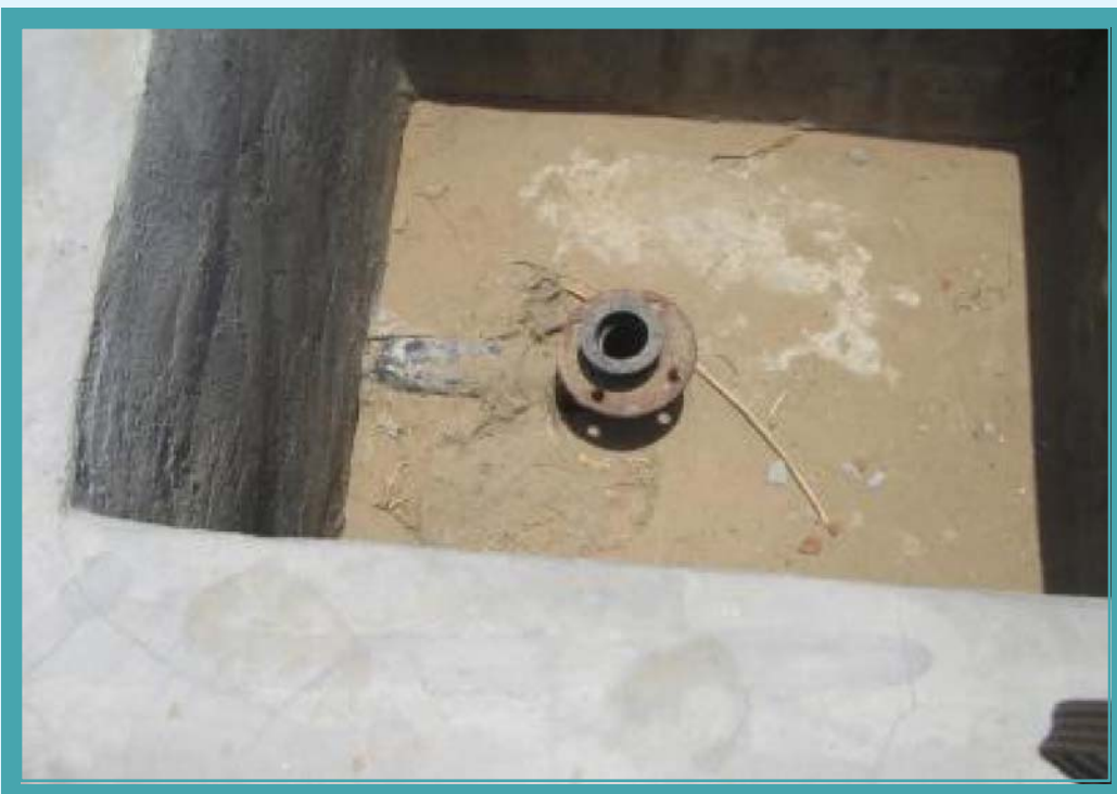
Narmada Canal Project – Incomplete work in the Inlet of Diggi No.5 Basan Minor at tail 3.701 km – Vank Distributary
