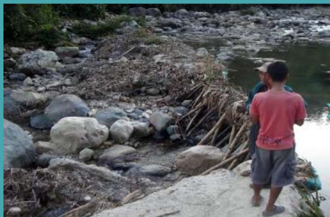
Damaged headwork and makeshift arrangements at Silte to Dekam MI Project at Ledum, Pasighat Division
