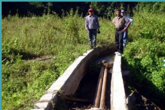
Damaged field channel in MI Project at Ganga Village, Itanagar Division
