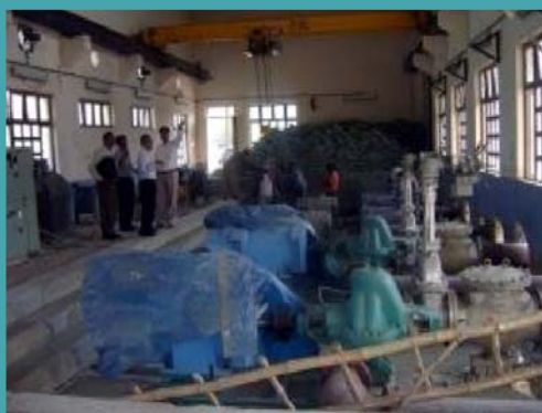
Pumping machinery for Zone 2A not functioning due to lack of power supply
