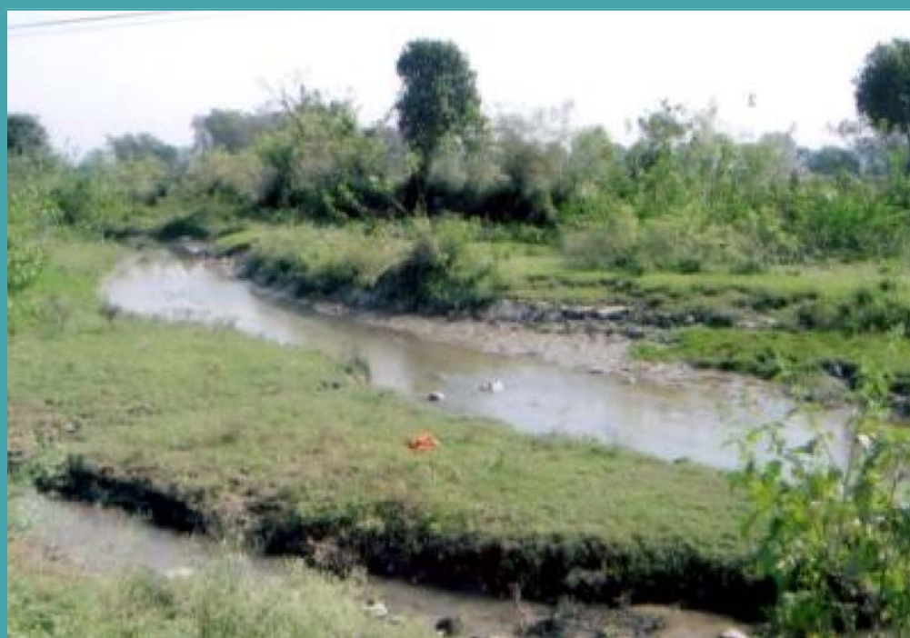
Unlined Portion of Basantpur Canal
