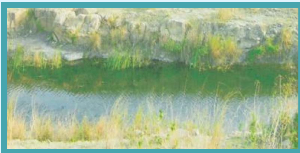
Right Bank Canal (RBC) of Rengali Irrigation Project (RIP) – Failure of slope and slippage of embankments at RD 34.24 km of RBC
