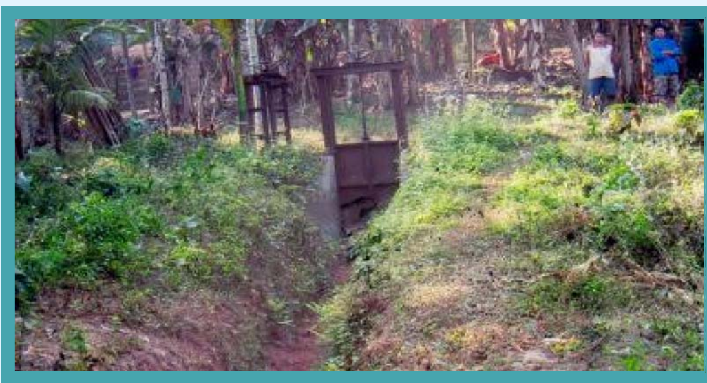
Gandual MI Project – Cross Regulator in the earthen canal with no water in the canal
