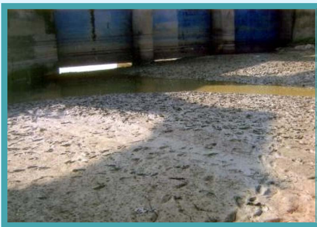
Siltation in upstream of Western Kosi Main Canal (WKMC) at RD 55 Km
