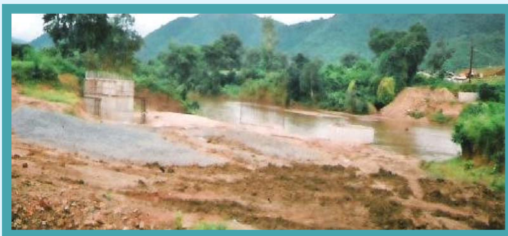
Upper Indravati Irrigation Project – Syphon Aquaduct over river Sagada at RD 2820 metre of REMC remained incomplete due to non finalization of design
