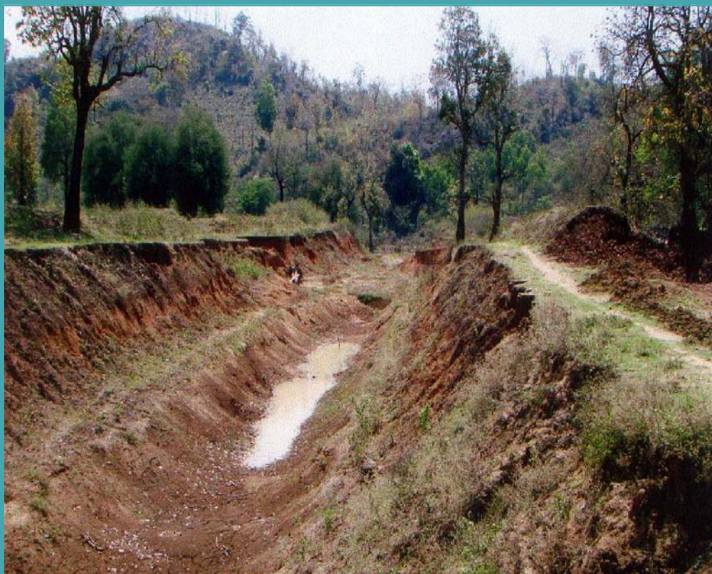
Doraguda MI Project – Incomplete Head reach canal from RD 00 metre to 1250 metre
