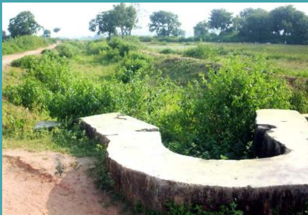
No water and need for bush clearing at Chainage 319 km of Tapkara Project
