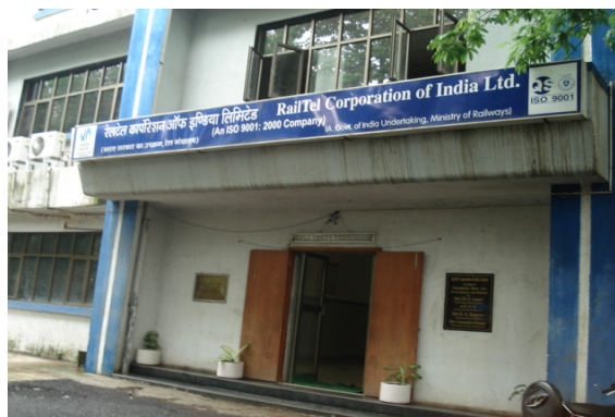
RCIL structure at Mahalaxmi, Mumbai
