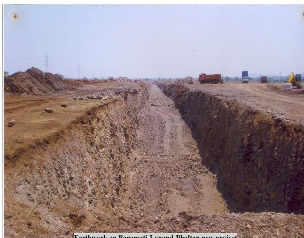
Earthwork on Baramati-Lonand-Phaltan new project
