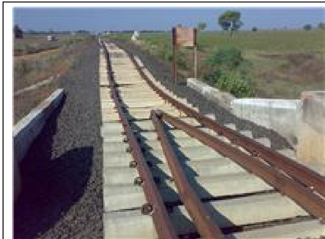
Amravati – Narkher New Lines Project (Sanctioned in 1993-94 – not yet completed)
