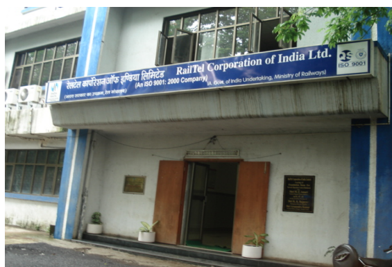
RCIL structure at Mahalaxmi, Mumbai
