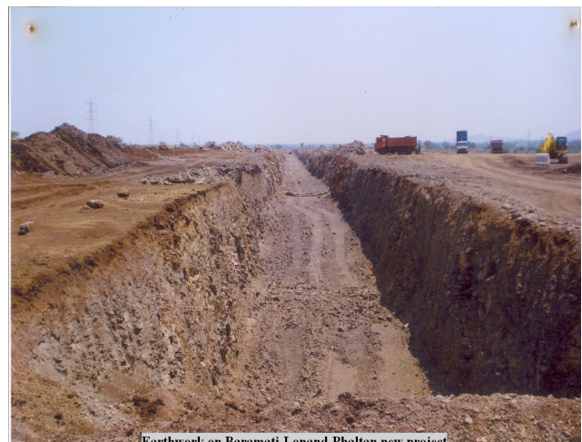
Earthwork on Baramati-Lonand-Phaltan new project
