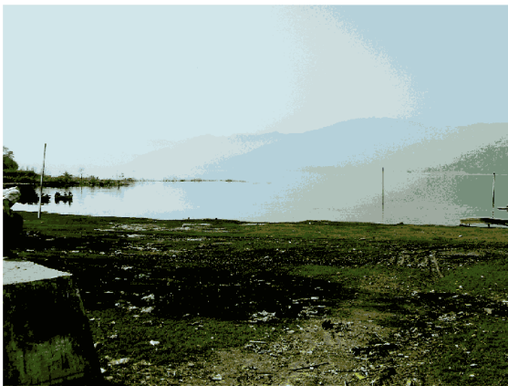
Jetty at Luhnu not constructed
