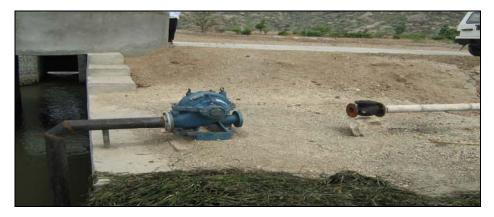
Photograph showing non-connection of rising main of water supply scheme with source (06.07.2010)
