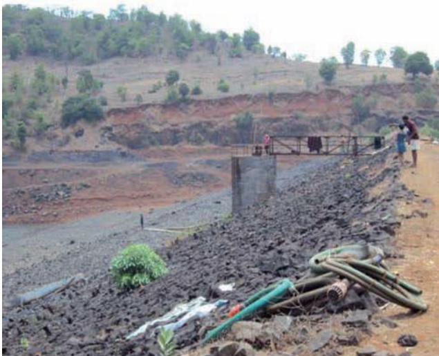
Tangar (leakage at dam flank)
