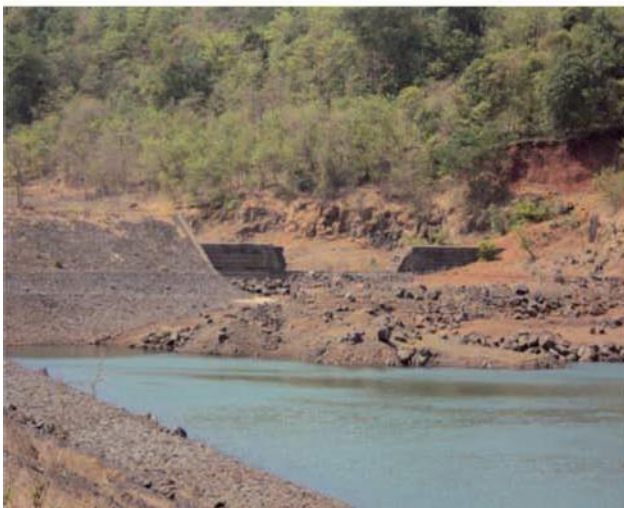
Kondivali (pilot cut in spillway)
