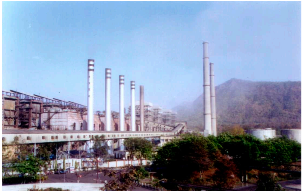
(Satpura Thermal Power Station, Sarni)
