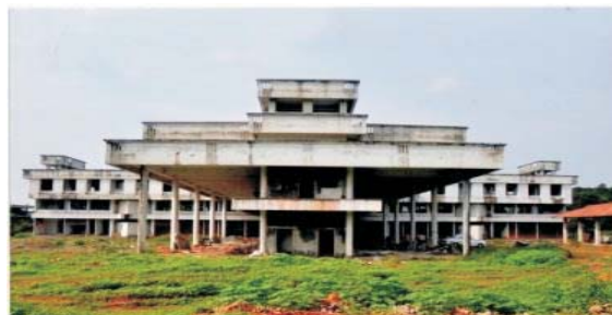
Bus terminal under construction
