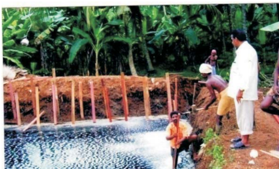
Leachate collected in temporary ponds
