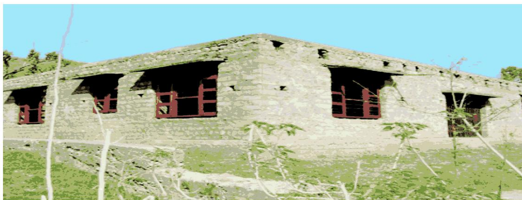
Incomplete Panchyat Ghar Jhanger
