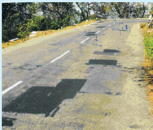
Mubarikpur-Ranital-Kangra road (km 117/635)
