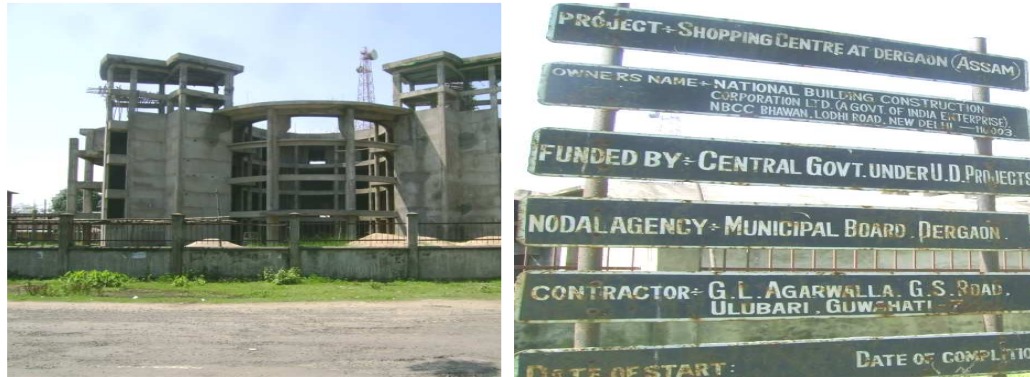
Market Complex at Dergaon constructed by NBCC (23 May 2010)
