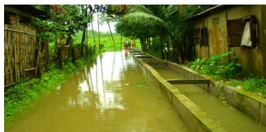
Storm water drainage at Karimganj town (2 June 2010)
