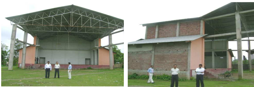
Community hall at Dergaon under SJSRY (cost- ₹35 lakh) (20 May 2010)
