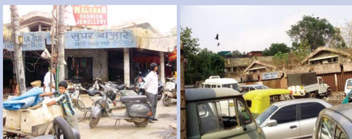
Dilapidated buildings in INA market
