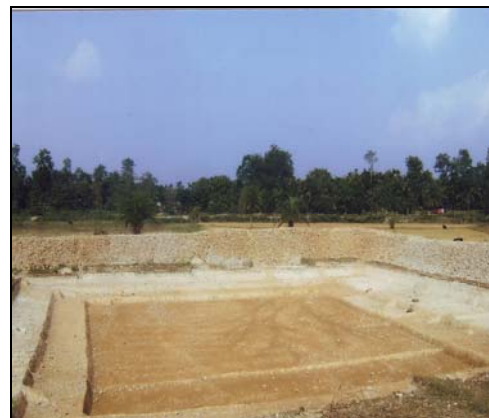
Construction of pond under Amarpur Nagar Panchayat
